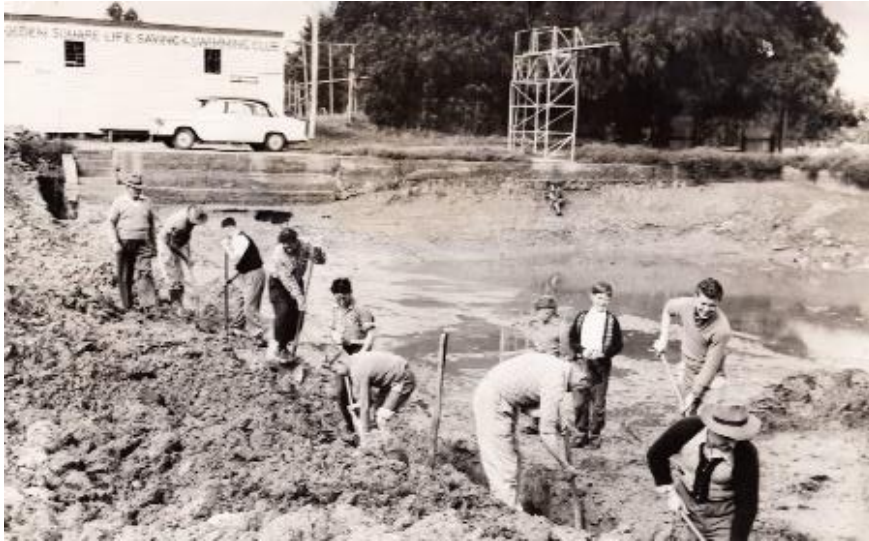
Digging out the pool for a concrete upgrade
